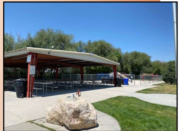
The bowery at Mountain View Park; this is one of many public facilities the city offers to residents.
